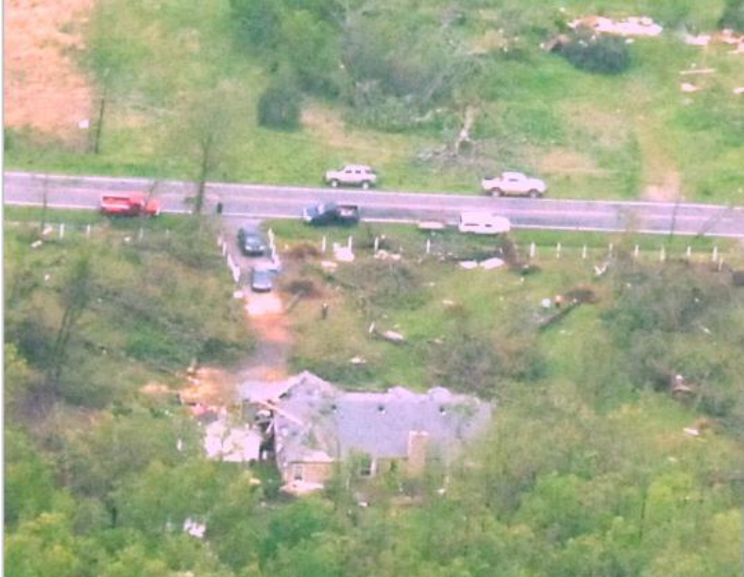
Figure 5.20 Minor damage to the residential house roof rated as EF1, R3L1 taken by CAP (2014).
