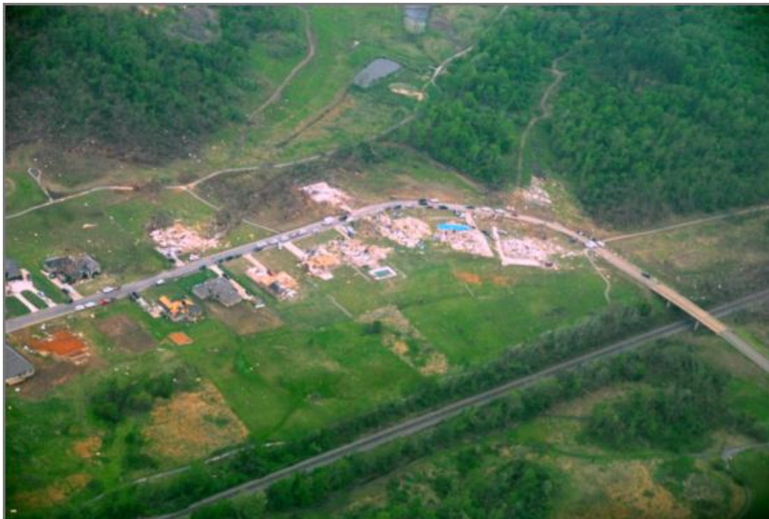
Figure 5.12 Severe damage in a community (R2L2) rated as EF4, taken by CAP (2014).
