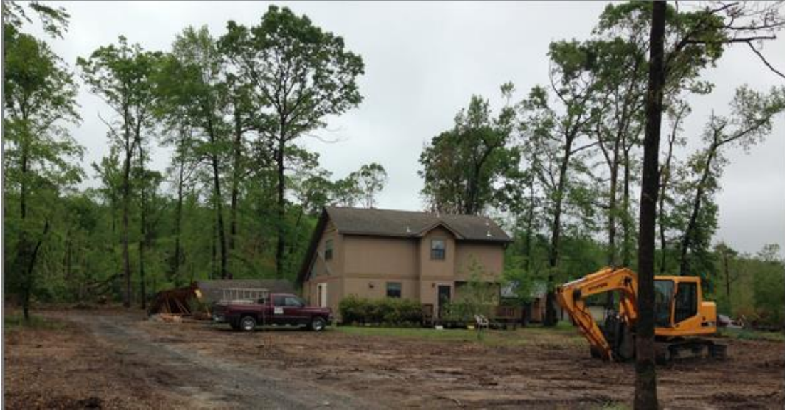
Figure 5.5 A house in location (R1L1) with a damage rating as EF1, only the shade attached to the house is collapse, taken by UA team.
