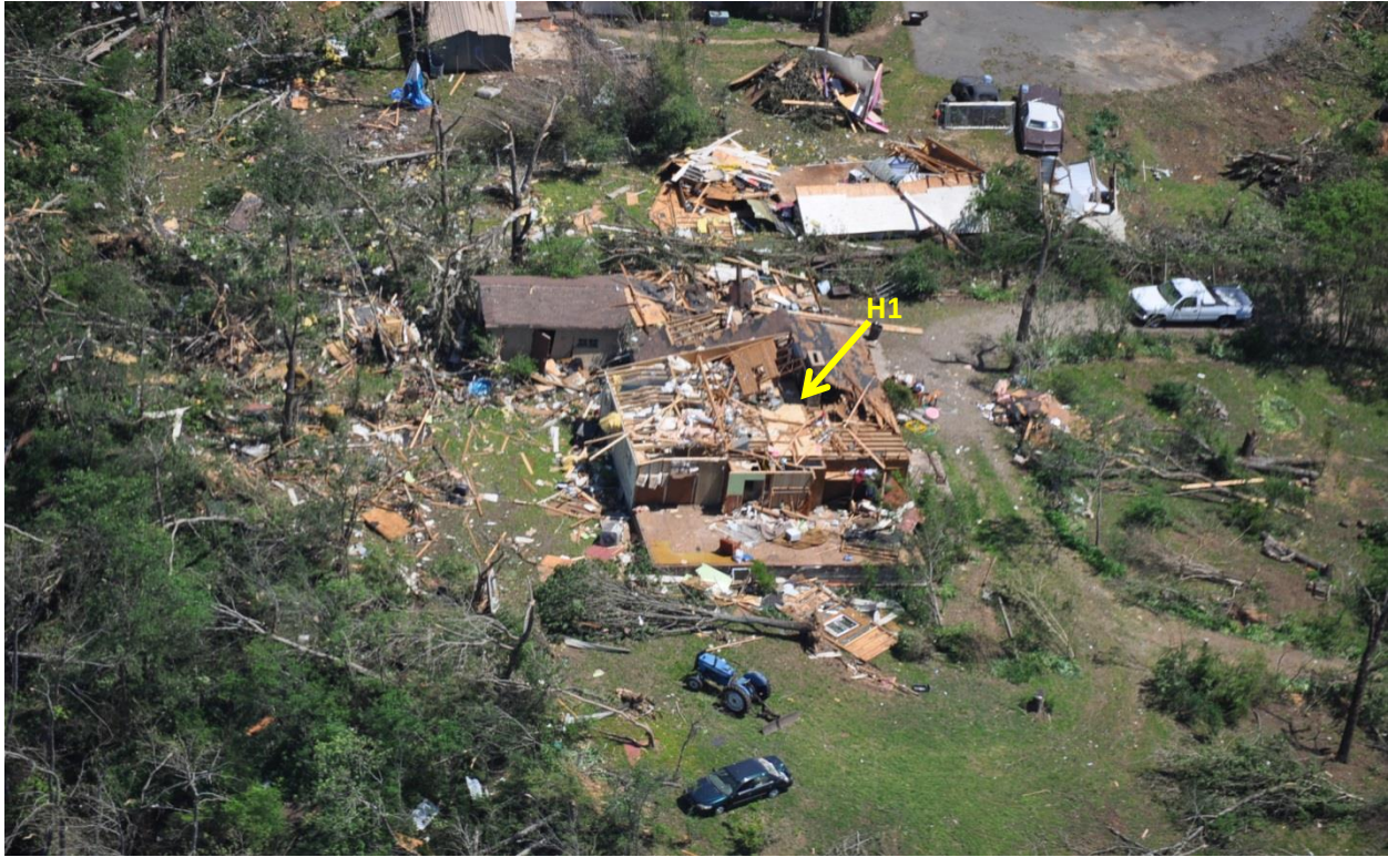
Figure 4.18 Aerial image for a severe damage for house (H1) uphill (Source CAP, 2014).
