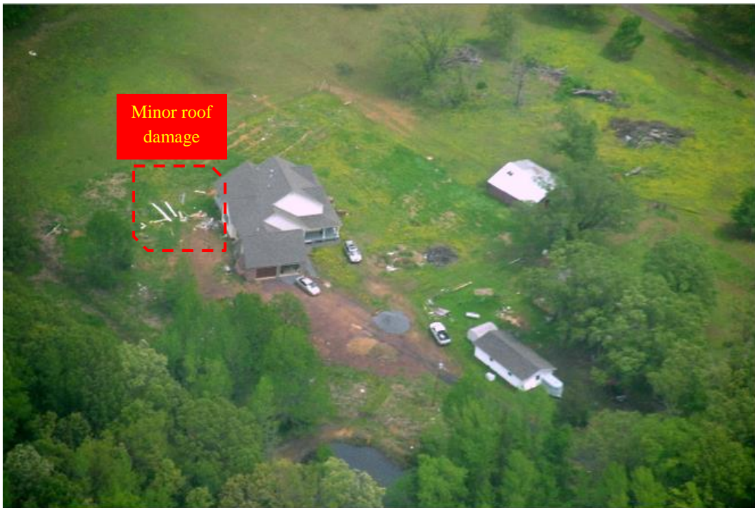
Figure 5.21 Minor roof damage rated as EF1, R3L1 taken by CAP (2014).
