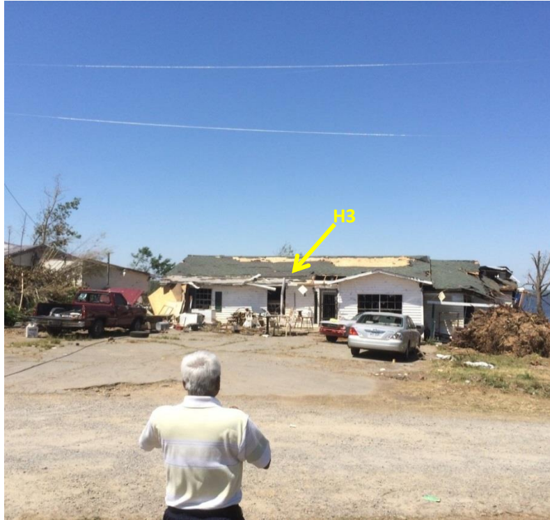
Figure 4.22 Minor damage (EF1) for the house (H3) on the leeward side (low elevation) (UA team photo).
