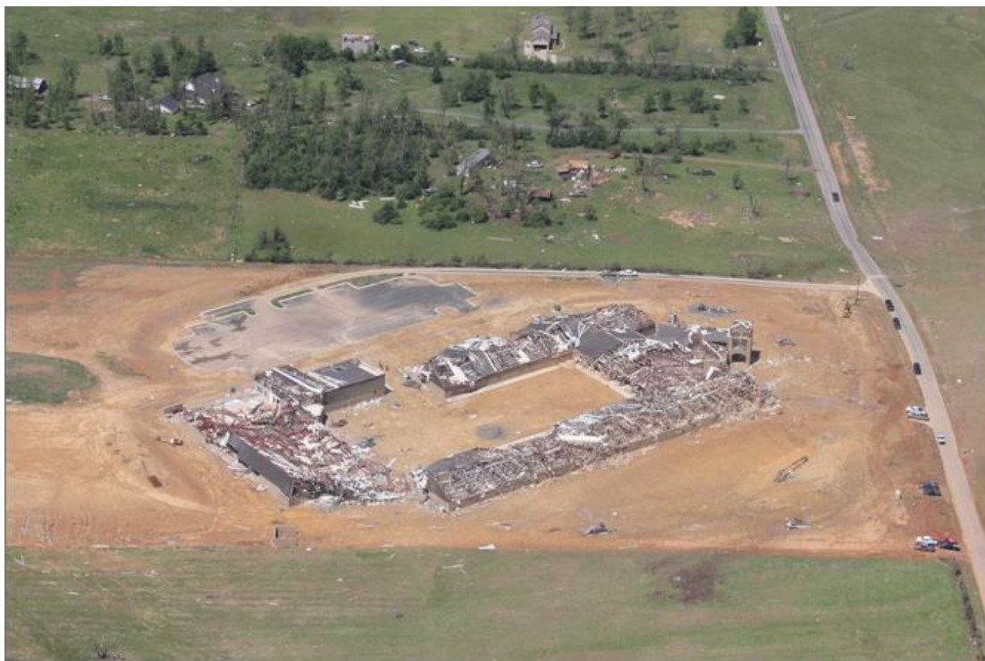
Figure 5.27 A new constructed school at location R4L1 heavily damaged and rated EF4, taken by CAP (2014).
