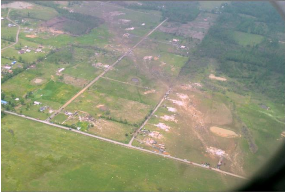
Figure 5.24 Several communities destroyed due to tornado right before Vilonia bypass at R3L2.
