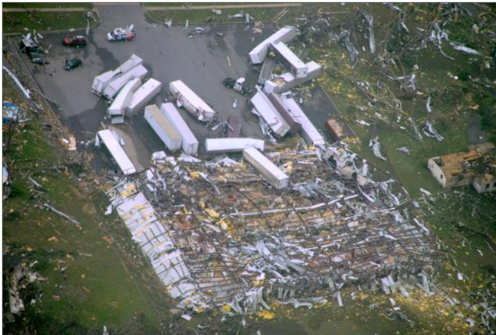
Figure 5.14 An aerial image for a metal building severely destroyed and rated as EF4 at location (R2L3), Taken by CAP (2014).
